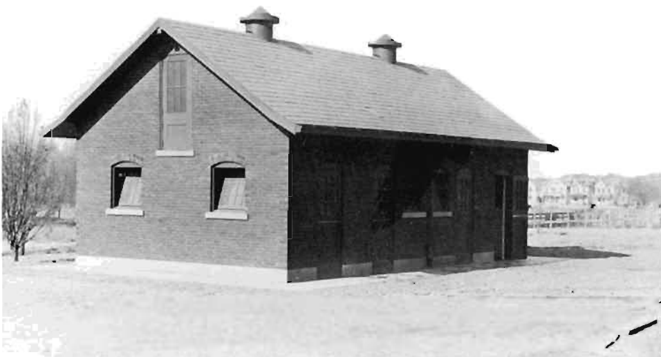
Left—The eight-stall Isolation Ward, built in 1910 to accommodate animals with infectious diseases.
