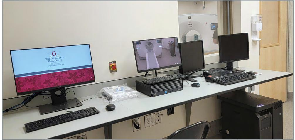
Within the control room, the computer fuses CT and PET images, with the CT providing anatomic resolution and the PET providing metabolic information.
