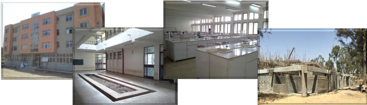
From left to right: The new Veterinary Academic building of the UoG Faculty of Veterinary Medicine, the new classroom building (which provides capacity to house all veterinary classes under one roof), one of the multiple teaching laboratories (in the picture the parasitology lab), and the new veterinary hospital currently under construction to be completed by 2017
